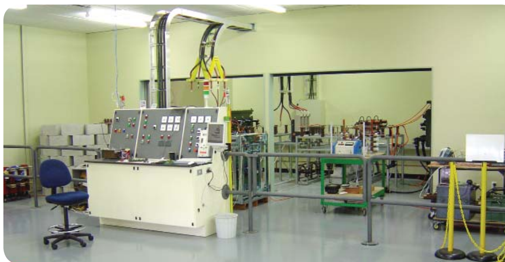
AuCom's medium voltage testing facility
